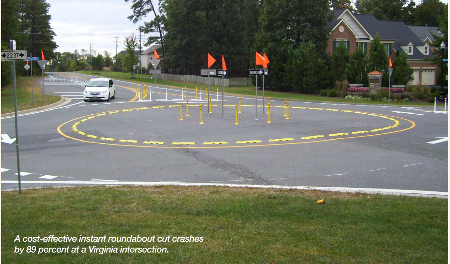
Credit: Virginia Department of Transportation
