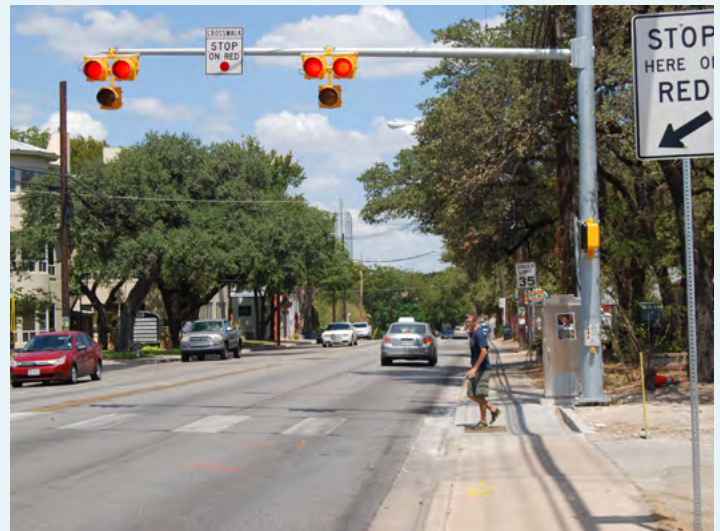
Pedestrian hybrid beacons enhance safety for walkers crossing multilane roads in Austin, TX.
